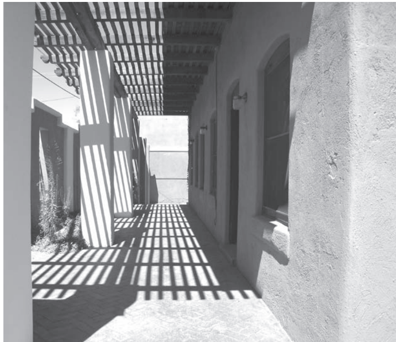
A view of our new headquarters at 300 N. Ash Alley, Tucson, Arizona, 85701. Stay tuned for details on the exciting transformation we have planned—and thank you for your support!
